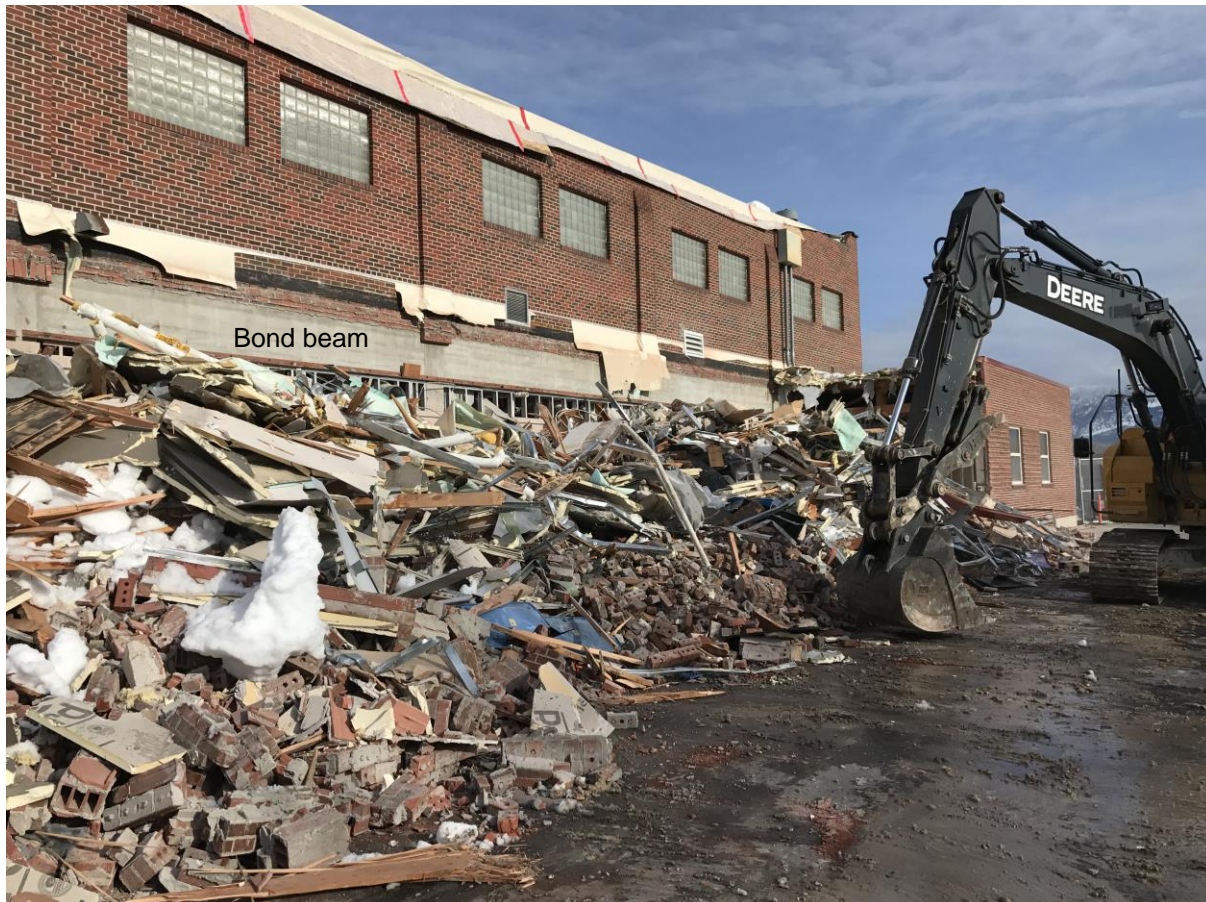
Locker rooms demolished
