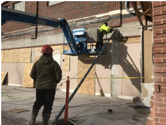
Swank installing bracing
