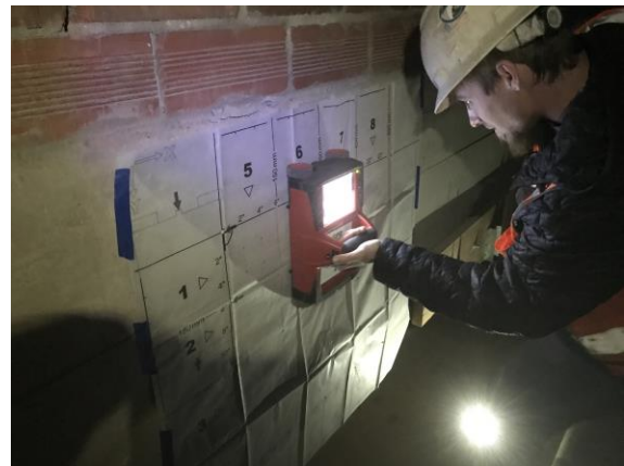
A-core scanning bond beam with GPR unit
